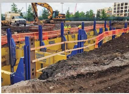
The Portable Construction Guardrail is designed to be used as a passive fall prevention barrier at leading edges or internal openings.
